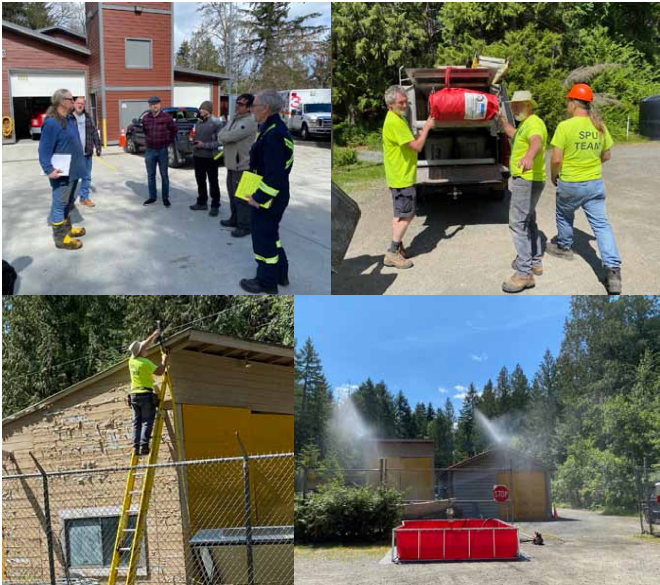
Upper left: pre-drill briefing. Upper right: loading the drop tank Lower left: installing the structure protection sprinklers. Lower right: drop tank feeding the sprinklers in action.
